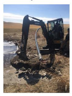
The DuPage Airport Authority completed a project to repair collapsed drainage pipe at the 4th hole tee complex. The repair corrected a low depressional area that was once continually flooded.
