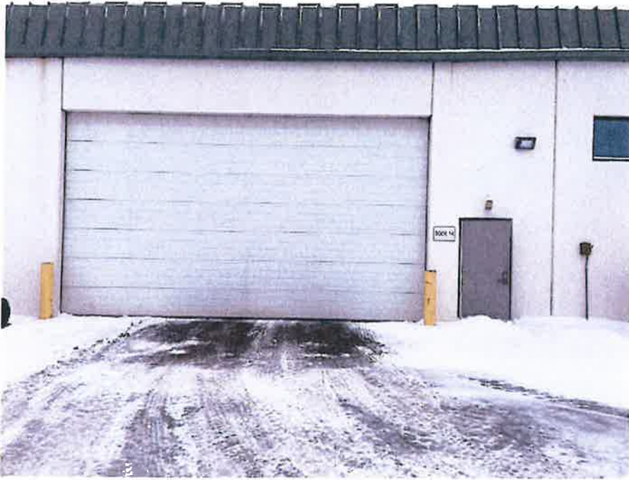
Existing Sectional Overhead Door
