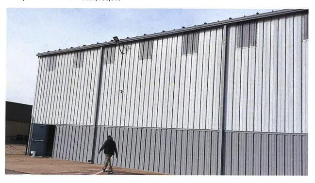
Exterior hangar façade renovations occurred at three (3) hangar locations. Renovations include caulking, painting, metal panel installation and gutter replacement. Completion is anticipated in April 2024. Total project cost is \$293,520.
