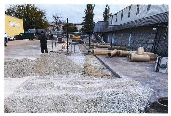
The Airport Authority completed a project to remove and replace failed drainage structures and pipe within the auto parking lot between Hangar E20 and E21 including associated paving work. Total project cost was \$143,544.
