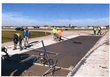
The Airport Authority completed a project to remove and replace several airfield concrete pavement panels, isolated drainage structures and hangar apron areas. Total project cost was \$385,088.
