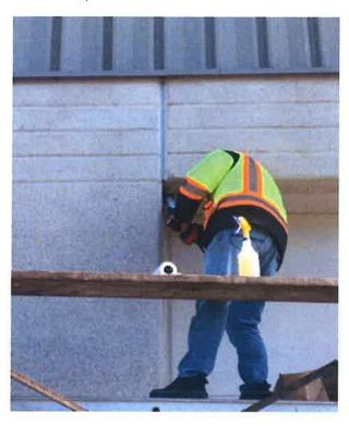
The Airport Authority completed a project to conduct exterior repairs to the N. Hightail and 1955 Aviation hangars. Repairs included caulking and patching, painting, sealing, new gutters and downspouts. Total project cost was \$529,861.
